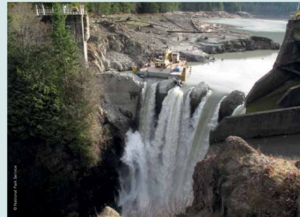
Removal of the Glines Canyon Dam on the Elwha River in 2014 (Washington state, USA), two years after removal of the Elwha Dam. These dams had caused a 99 percent reduction in the Elwha's salmon numbers, previously upwards of 400,000 per year across five species of salmon. The combined capacity of the two dams was 28 MW; since dam removal began, Washington State has added nearly 1000 MW of wind power.
